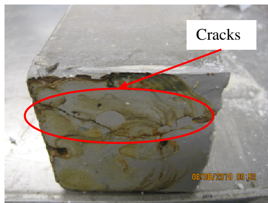
Figure 4.8. Cracks on specimen SP1-CI-13
