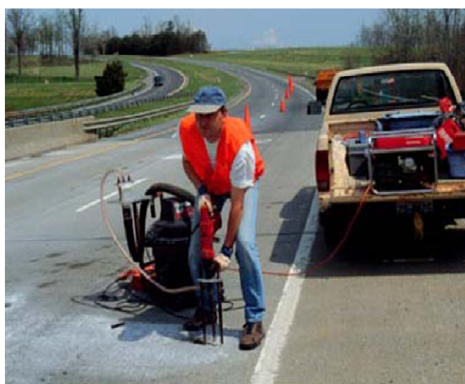
Figure 2.7. Sampling for chloride concentrations – collection apparatus: impact drill with hollow drill bit, powder concrete collection unit, and vacuum (Zemajtis 1998)
